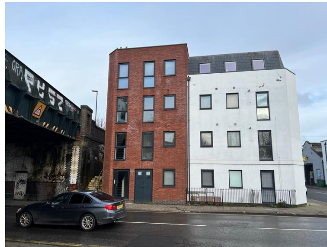
453 High Street (opposite the site)
